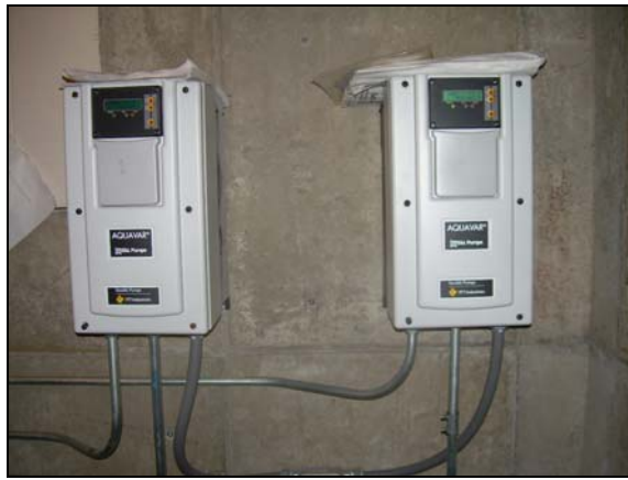
Photo #10 – Variable Speed Drives at Poker Hill Booster Station
