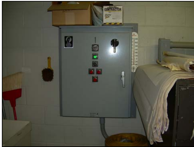
Photo #16 – Well Pump #1 Controls
