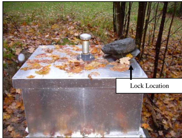
Photo #4 – Cistern Hatch & Vent
