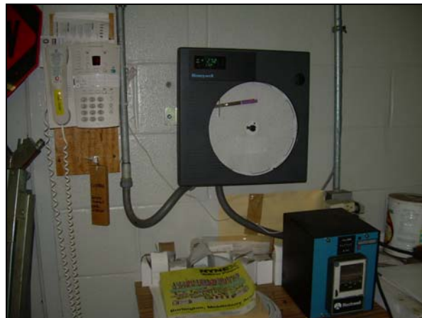
Photo #18 – 2-pen Chart Recorder (Tank Levels)
